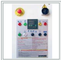
Electromechanical control panel.
