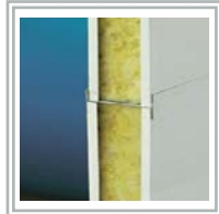
Dual skin wall panels joined by H channels with rock-wool insulation.
